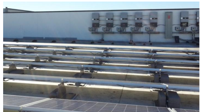
Parapet wall installation < 10ft boundary
