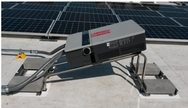
Low tilt angle installation < 10ft boundary
